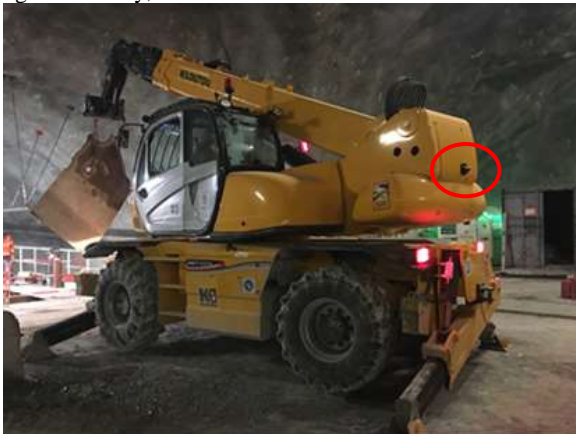
Figure 9: video-camera system installed on wheeled mobile crane.
