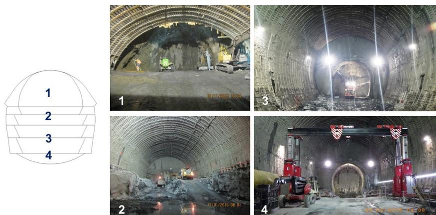
Fig. 7. Cross section of the the Assembly Cavern with photographs illustrating the excavation and construction stages in sequence 1, 2, 3 and 4.
