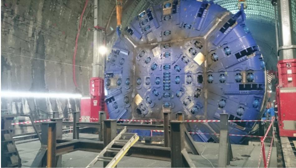
Fig. 9. The TBM head during assembling and lifting.
