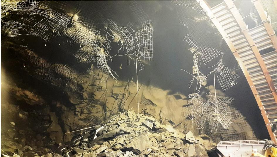
Fig. 8. Local instability at the right sidewall during excavation of the top heading.
