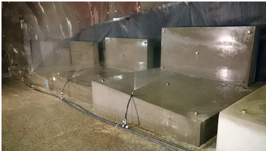
Figure 5. Test blocks in place with the sealed tacheometric monitoring marks
