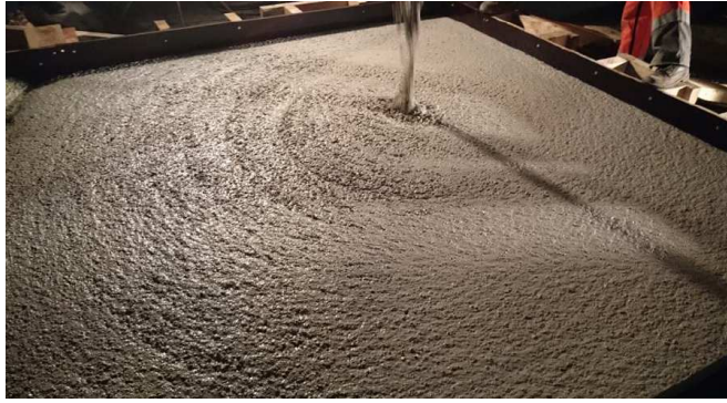
Figure 3. End of casting of the slab after placing the welded mesh
