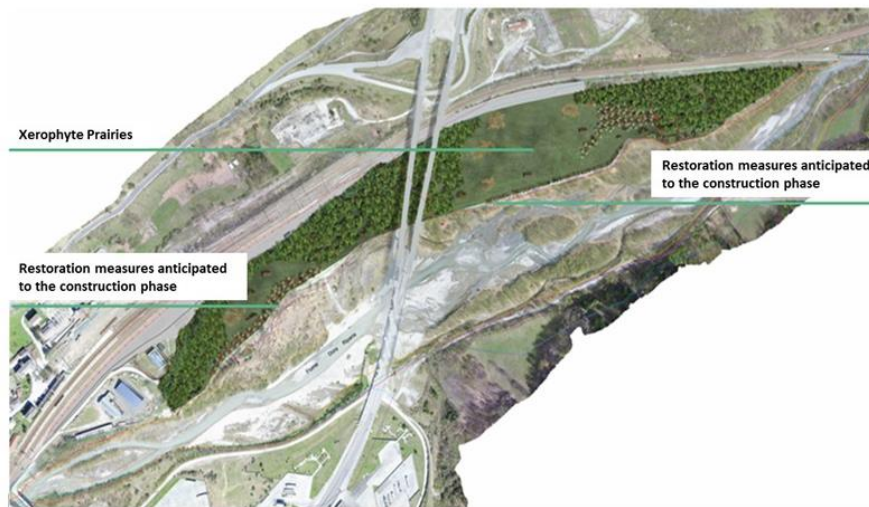
Figure 6. Restoration activities and final development of the Salbertrand construction site
