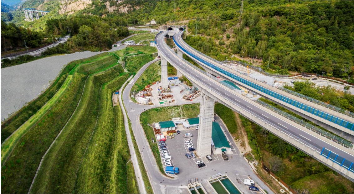
Figure 3. The Maddalena reconnaissance tunnel construction site
