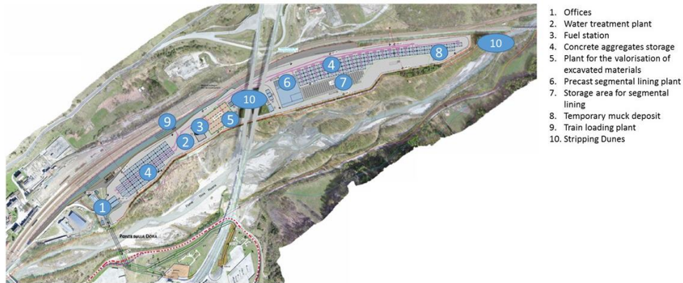
Figure 5. The Salbertrand Industrial Construction Site
