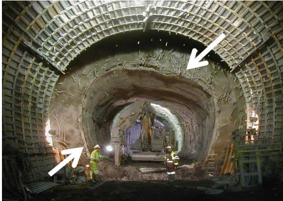
Figure 2. Convergence problems encountered in the Saint-Martin-la-Porte access tunnel.
